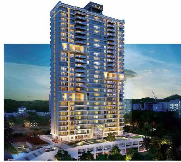
VIRAJ TOWER 4BHK, 5BHK Pokharan Road No. 2, Thane (W)
