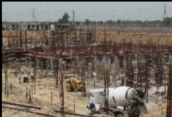
Atharva - construction photograph
