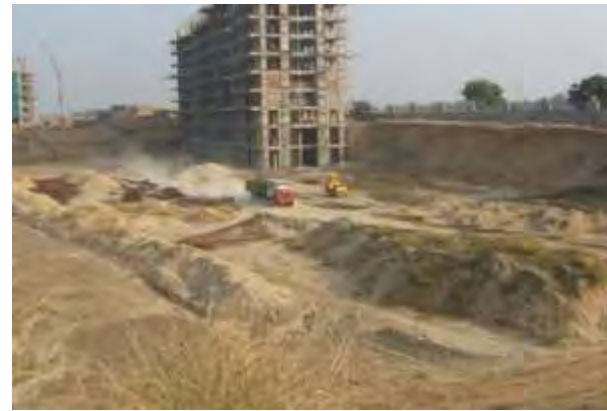
Sampada - development activities started
